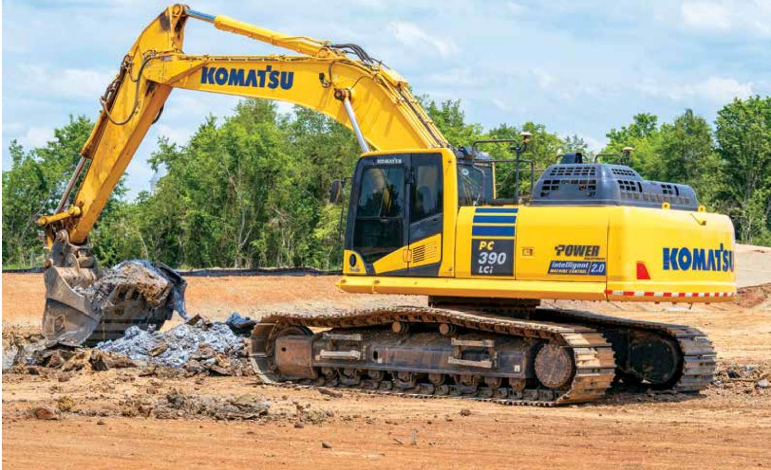
L&L Contracting relies on its Komatsu PC390LCi-11 IMC excavator to load trucks and maintain production during remediation work at a 22-acre big-box retail site in Alcoa, Tennessee.
