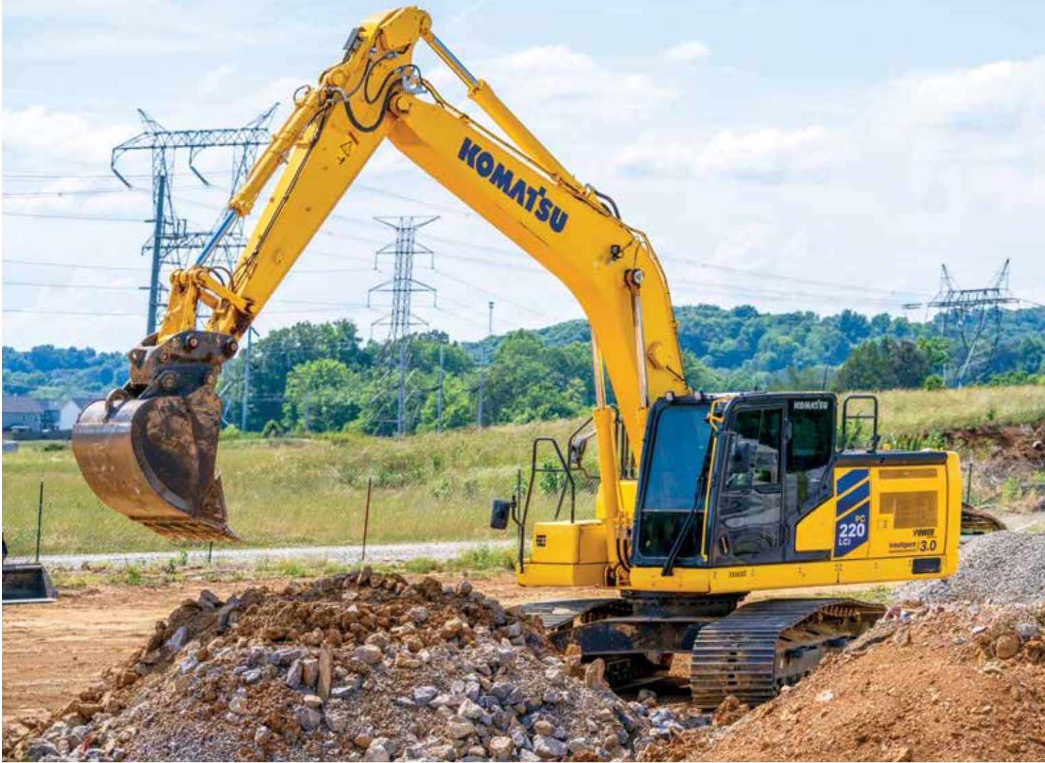
L&L Contracting uses its new Komatsu PC220LCi-12 intelligent machine control (IMC) 3.0 excavator for underground utility work, where IMC helps operators maintain grade and create as-builts.
