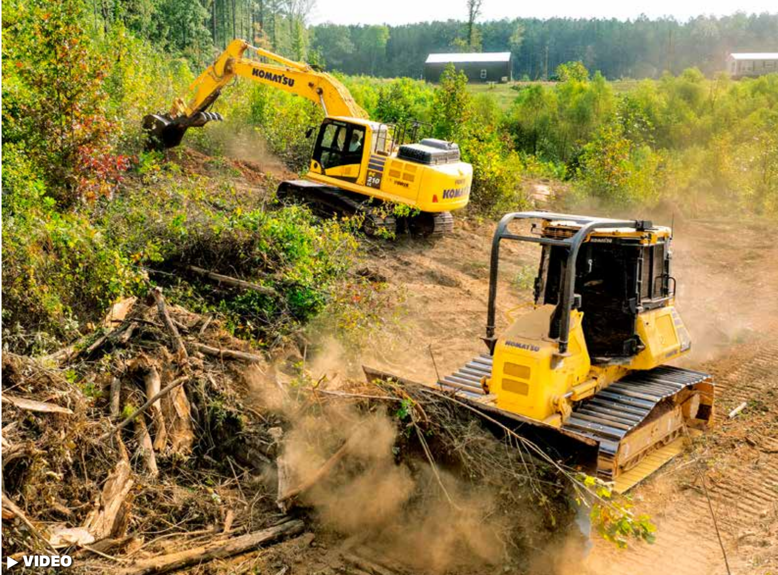
ZSD uses its Komatsu PC210LC-11 excavator and Komatsu D51PX-24 dozer in tandem to remove and pile material during clearing.
