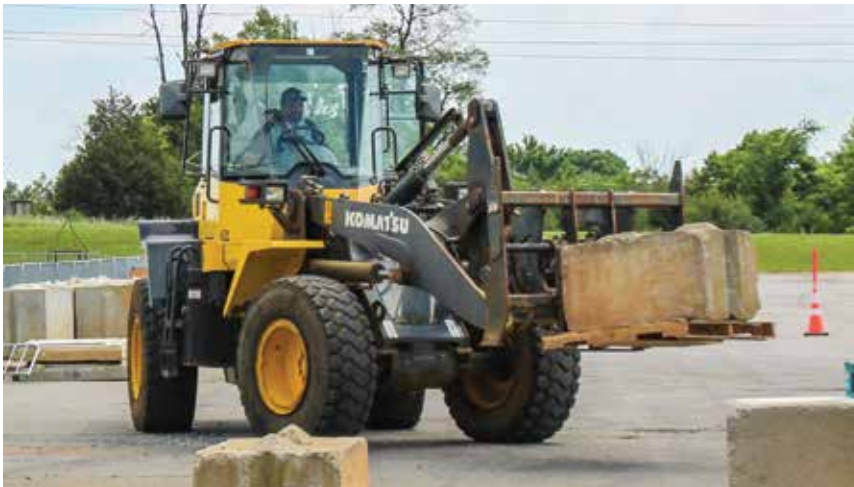
An operator transports material with a Komatsu WA200 wheel loader.
