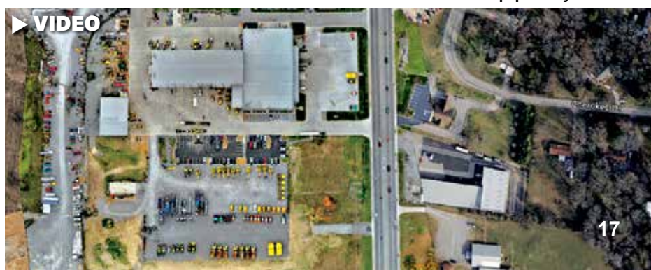
Power Equipment Company's Nashville branch renovations include expanded parking and a larger equipment yard.
